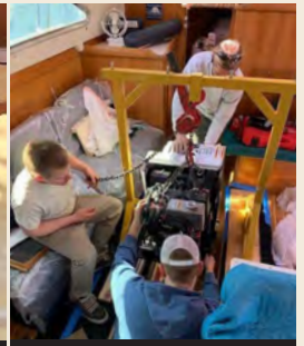
GENERATOR INSTALL
